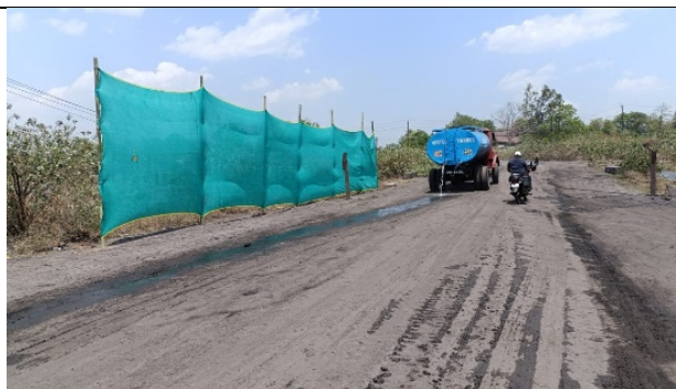
(Water Sprinkling from Mobile Tanker)
