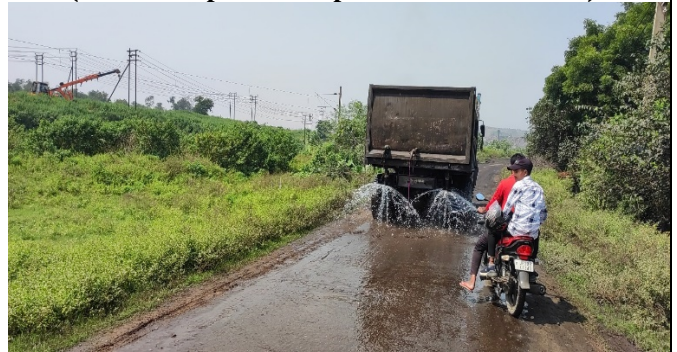
(Water Sprinkling from Mobile Tanker)
