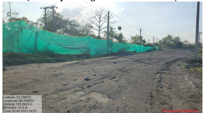
(Wind barrier on Moonidih washery road)
